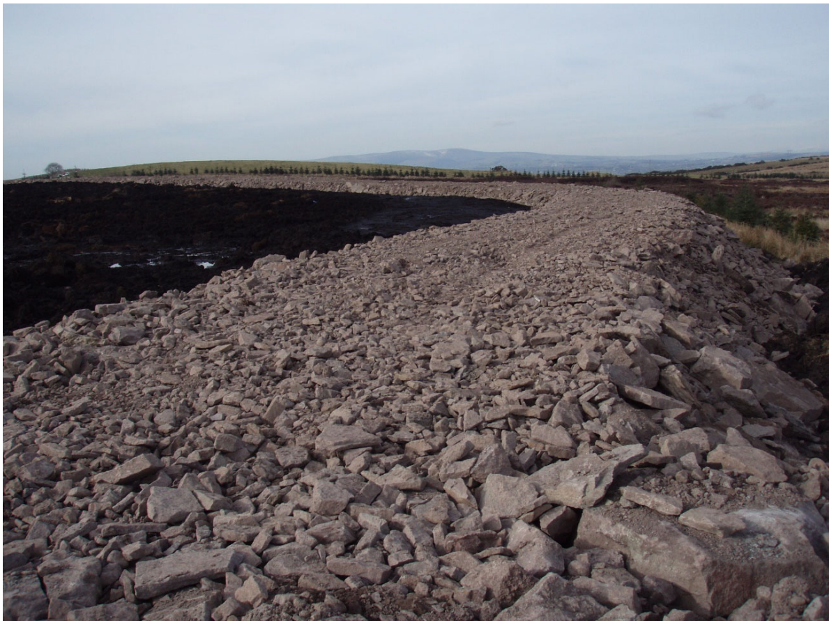
Photo 4 – Bunded peat repository site on the Crockagarran Wind Farm, Co. Tyrone
