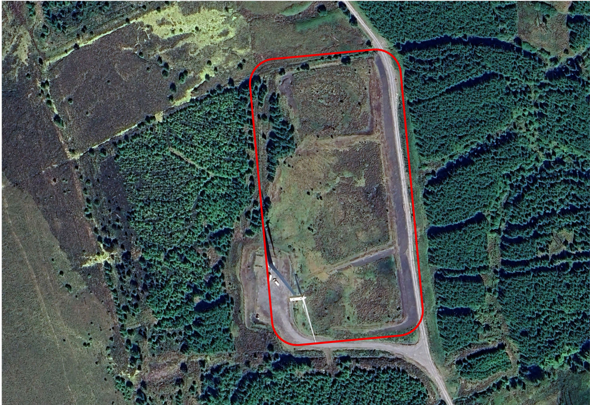
Photo 5 – Recent aerial photo of bunded peat repository cells on the Garvagh Glebe Wind Farm.
